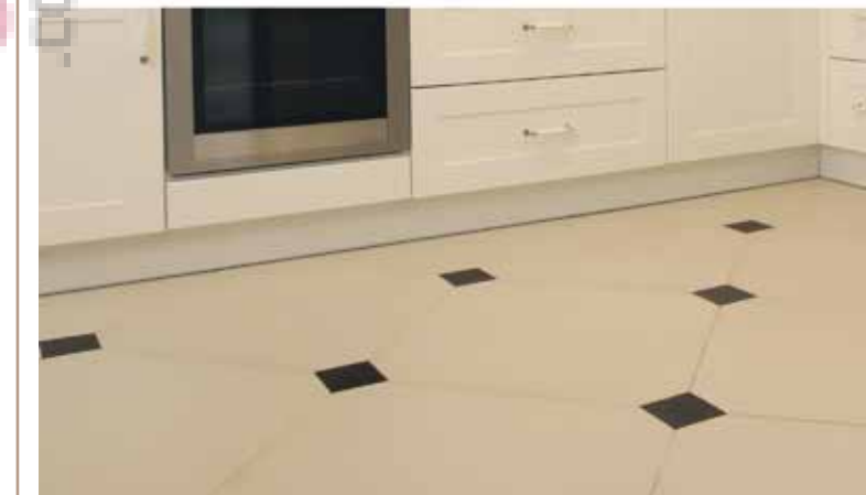
L-shaped kitchen platform, Vitrified flooring & Stainless steel sink
